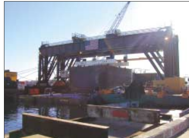
Catamaran barge/lifting beams supporting Box 15 prior to transport to cofferdam.
