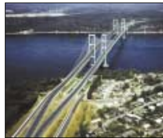
When it opens in 2005, the new crossing will parallel the existing one, which opened in 1950.
