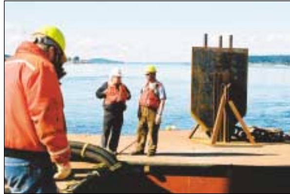
Driven Plate Anchor.
