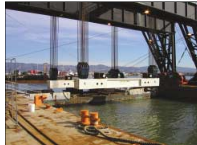
Catamaran barge/lifting beams picking Box 15 off of the transport barge.
