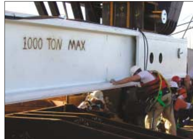
KFM workers connect lifting beam to Box 15 eyepads.
