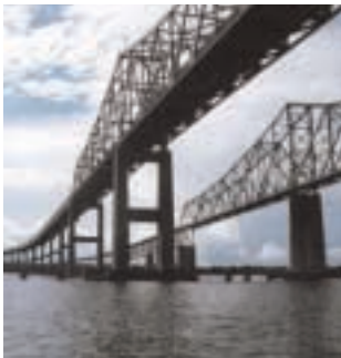
Existing Grace Memorial Bridge
