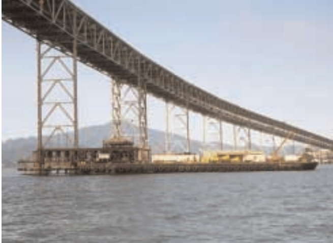
Richmond-San Rafael Bridge
