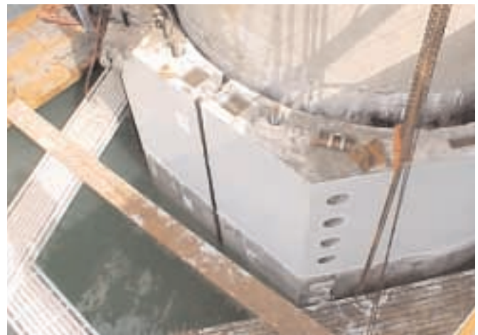
Precast Jacket Construction from Field
