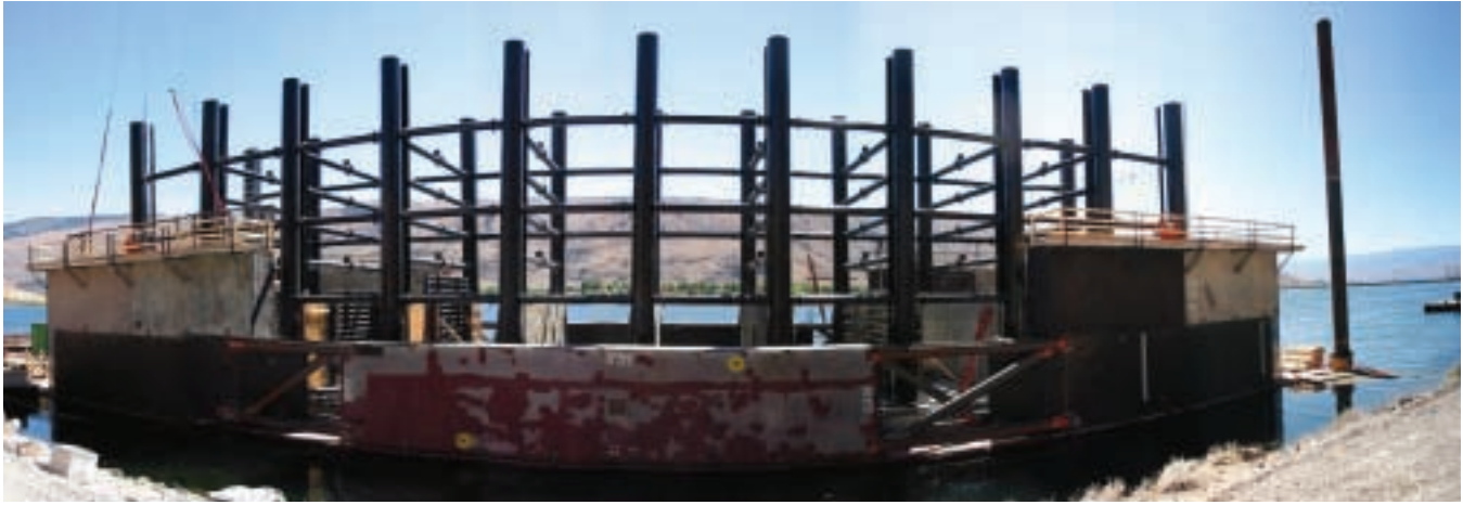
Pump Station Substructure on Casting Barge
