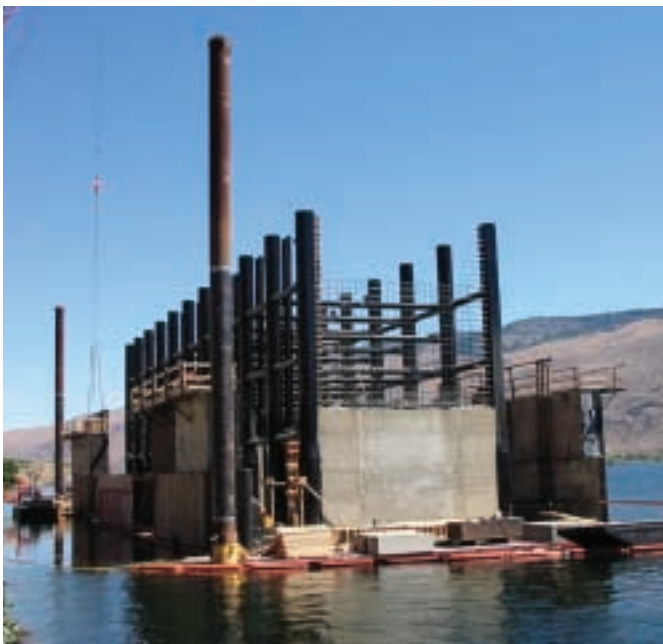
Casting of Concrete and Walls
