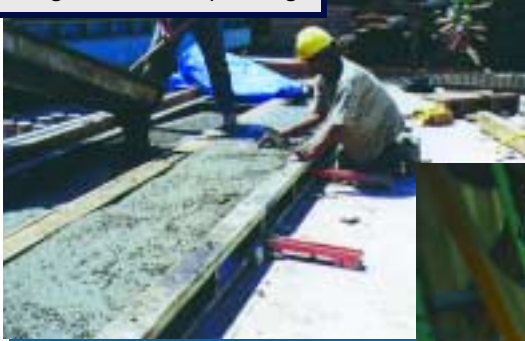
Finishing of self compacting
