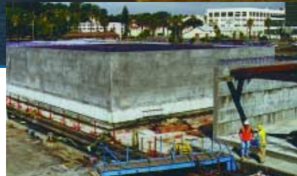
Interior of completed float-in cofferdam
