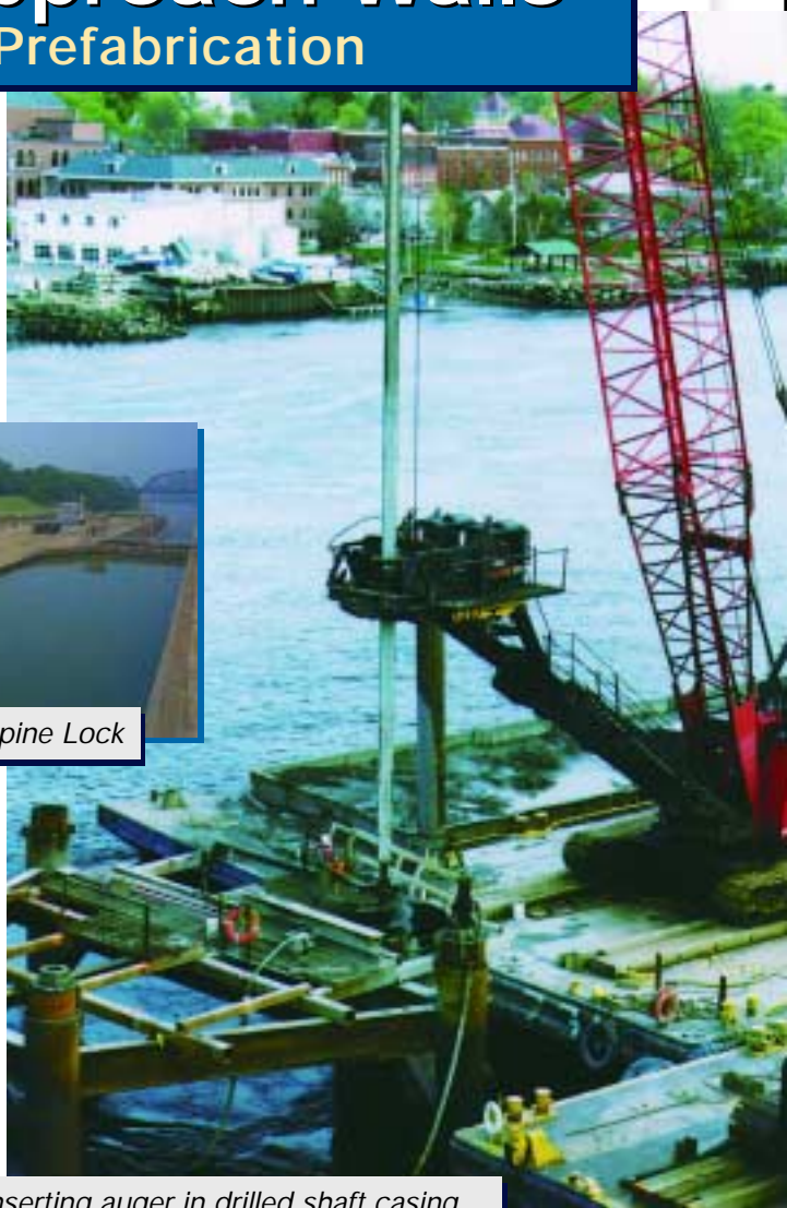
Inserting auger in drilled shaft casing
