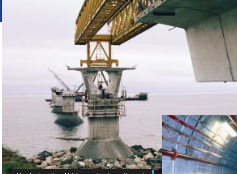
Confederation Bridge in Eastern Canada
