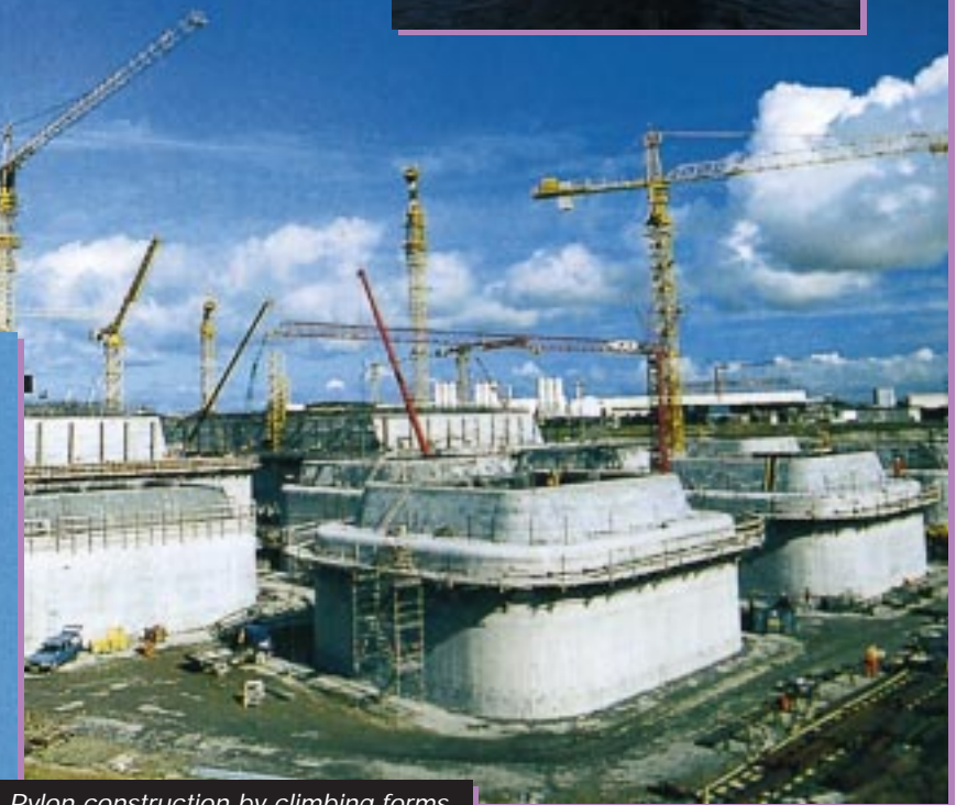
Pylon construction by climbing forms
