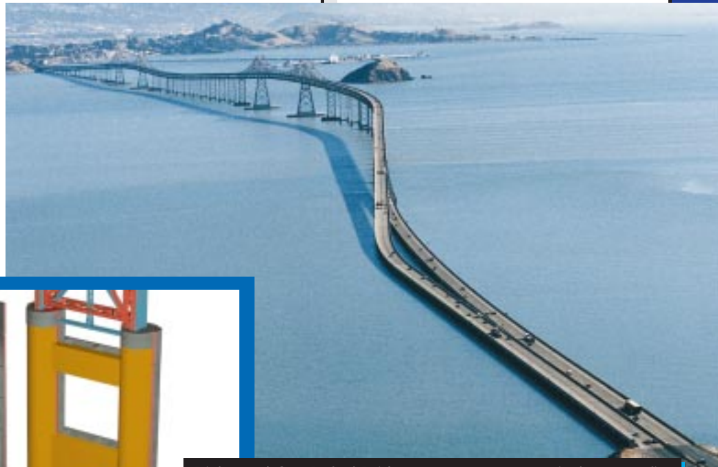
Richmond-San Rafael Bridge – precast concrete jackets retrofit
