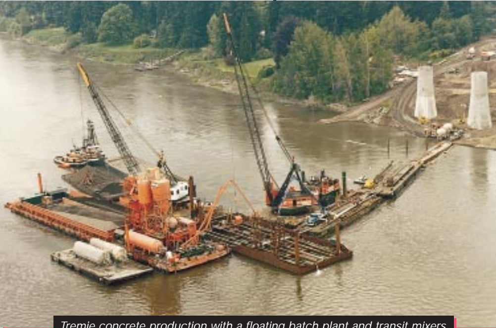
Tremie concrete production with a floating batch plant and transit mixers
