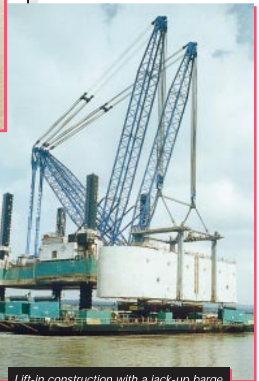
Lift-in construction with a jack-up barge
