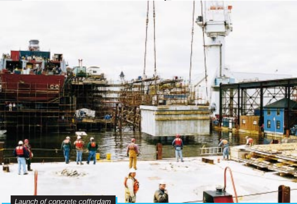
Launch of concrete cofferdam
