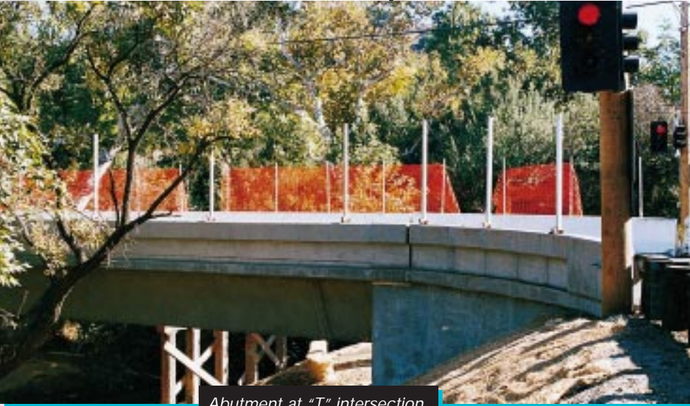
Abutment at "T" intersection
