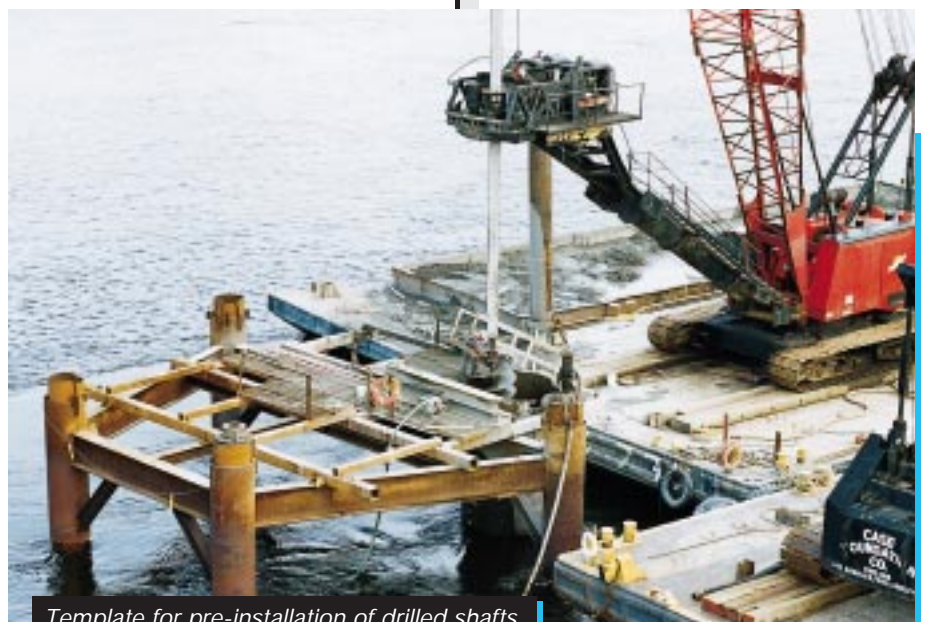
Template for pre-installation of drilled shafts
