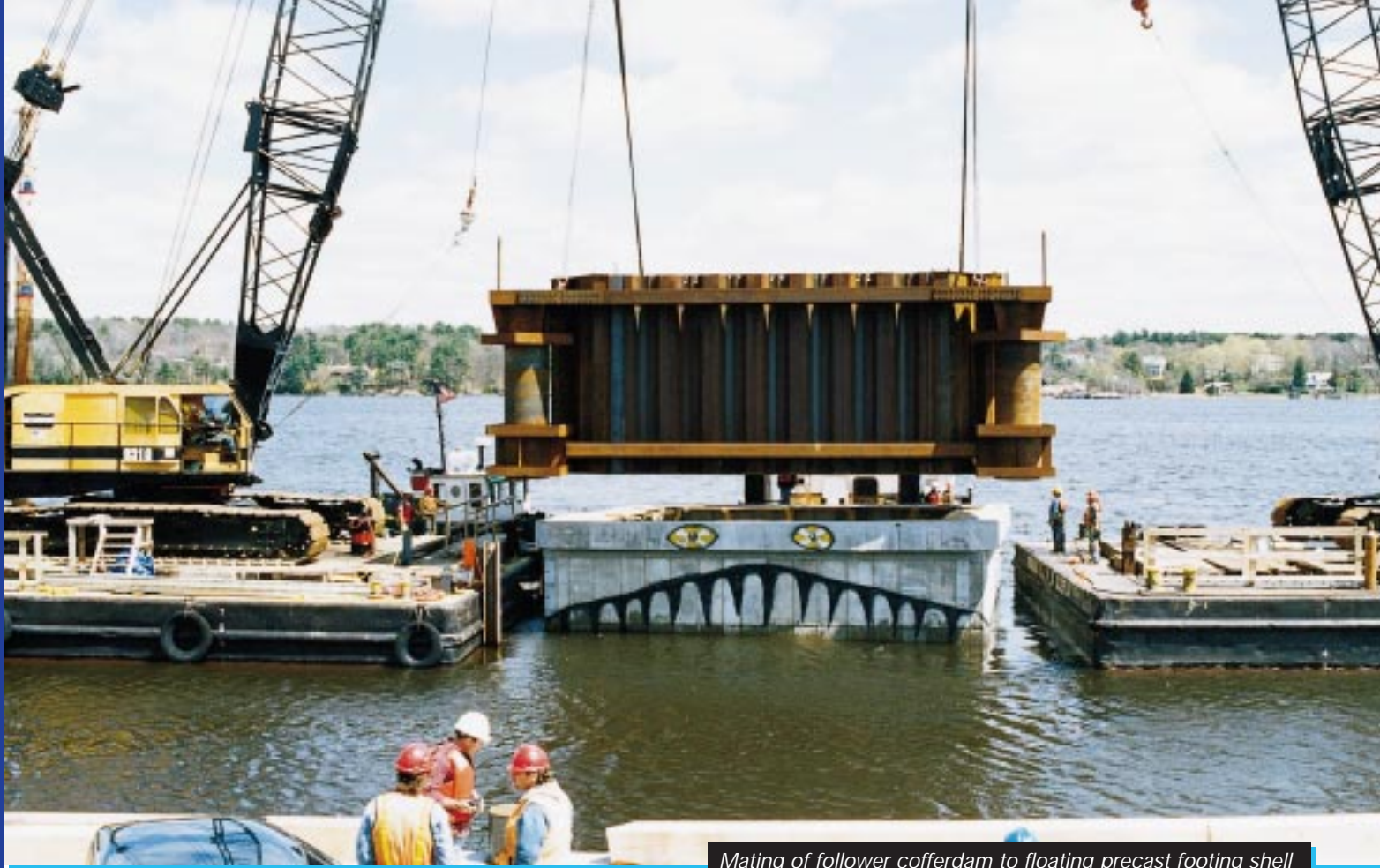
Mating of follower cofferdam to floating precast footing shell
