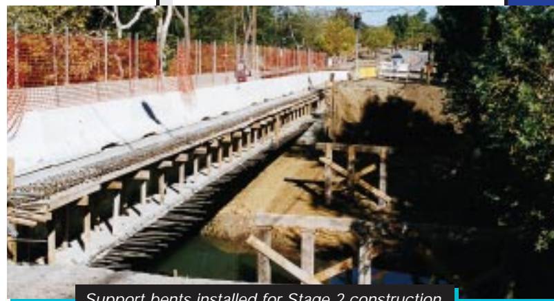
Support bents installed for Stage 2 construction
