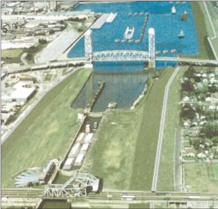
IHNC Lock under construction
