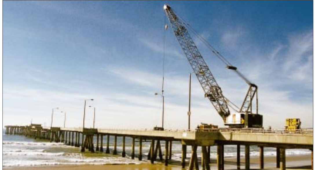
South side of existing pier.
