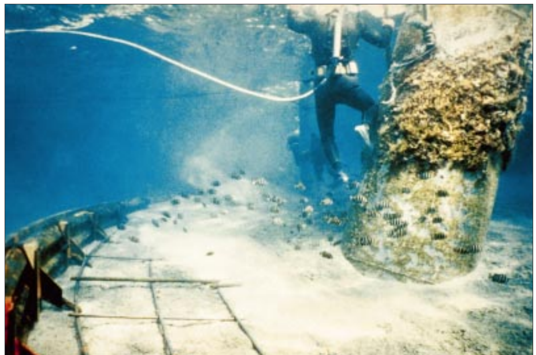
Placement of high quality underwater concrete leaving the marine life undisturbed.
