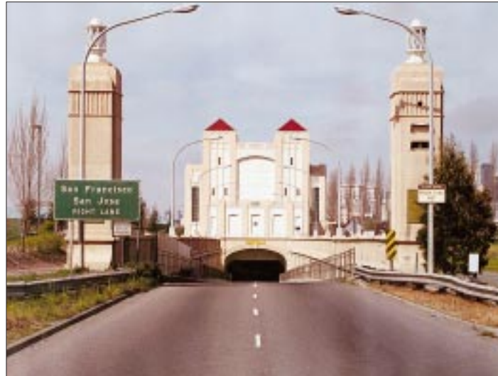
Alameda entrance to the Posey St. Tube.
