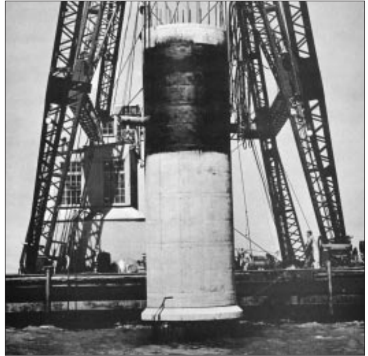
Placing existing precast shaft.
