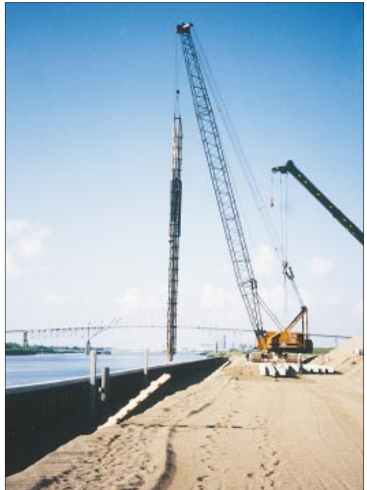
Driving relieving platform piles.
