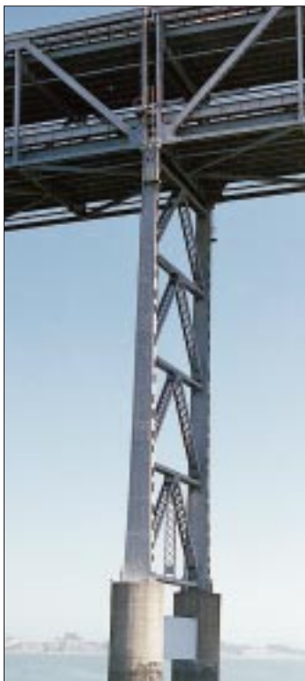
Typical two-legged tower.
