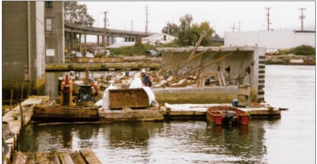
Precast concrete fender walls with temporary braces to concrete deck.
