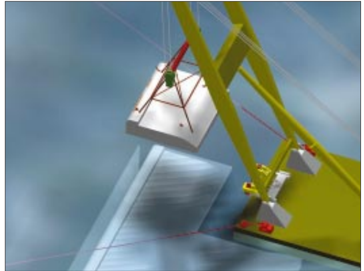
Illustration of precast concrete shell placed for Olmsted Dam.
