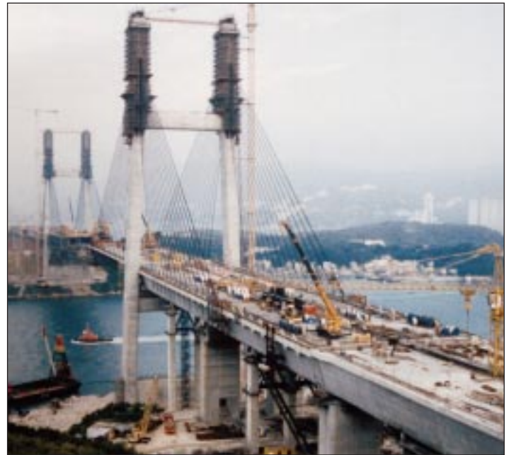
Kap Shui Mun Bridge in final stages of construction.
