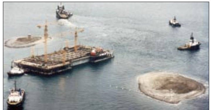
Deployment by floating technique of anchorblock caisson.
