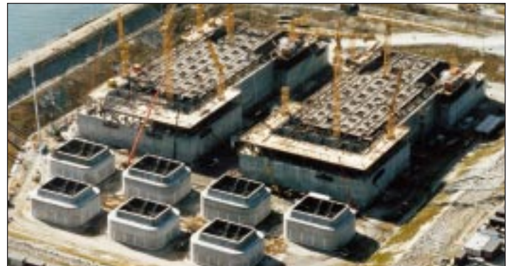
Drydocks for caisson construction up to 50,000t.
