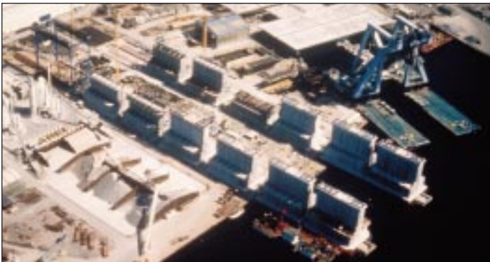
Precasting of West Bridge units on skidways.
