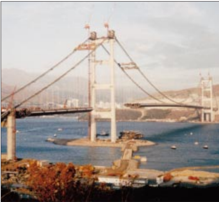
Tsing Ma Bridge nearing completion.
