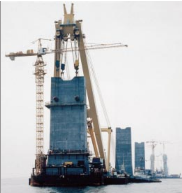
View of heavy-lift crane moving precast element.
