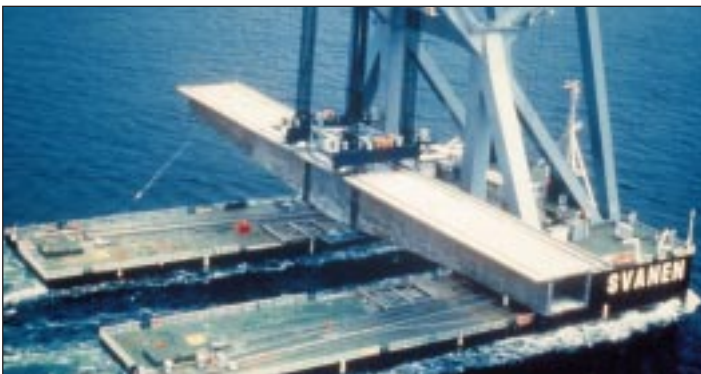
Deployment of precast superstructure unit by crane barge.
