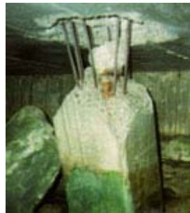
Section of upgraded Berth 40
