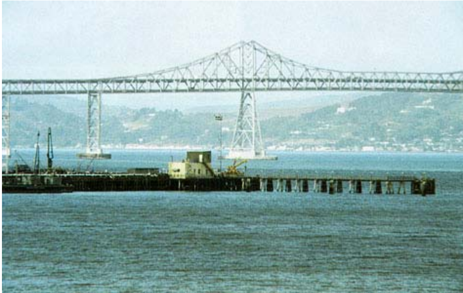
Point Molate existing Fuel Pier near Richmond-San Rafael Bridge.
