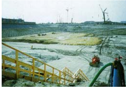
Drydock for construction of anchor block caissons
