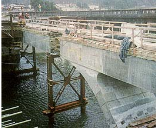
Approach span under construction next to badly corroded old bridge.
