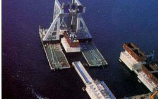
The "Swan" Lifting Foundation caisson for journey to the prepared seabed.
