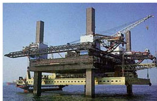
The "Buzzard" in position for seabed preparation for the foundation caissons.
