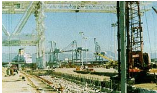
7th Street Terminal rehabilitation works.
