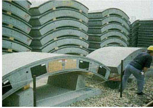
Prefabrication plant for tunnel lining segments.
