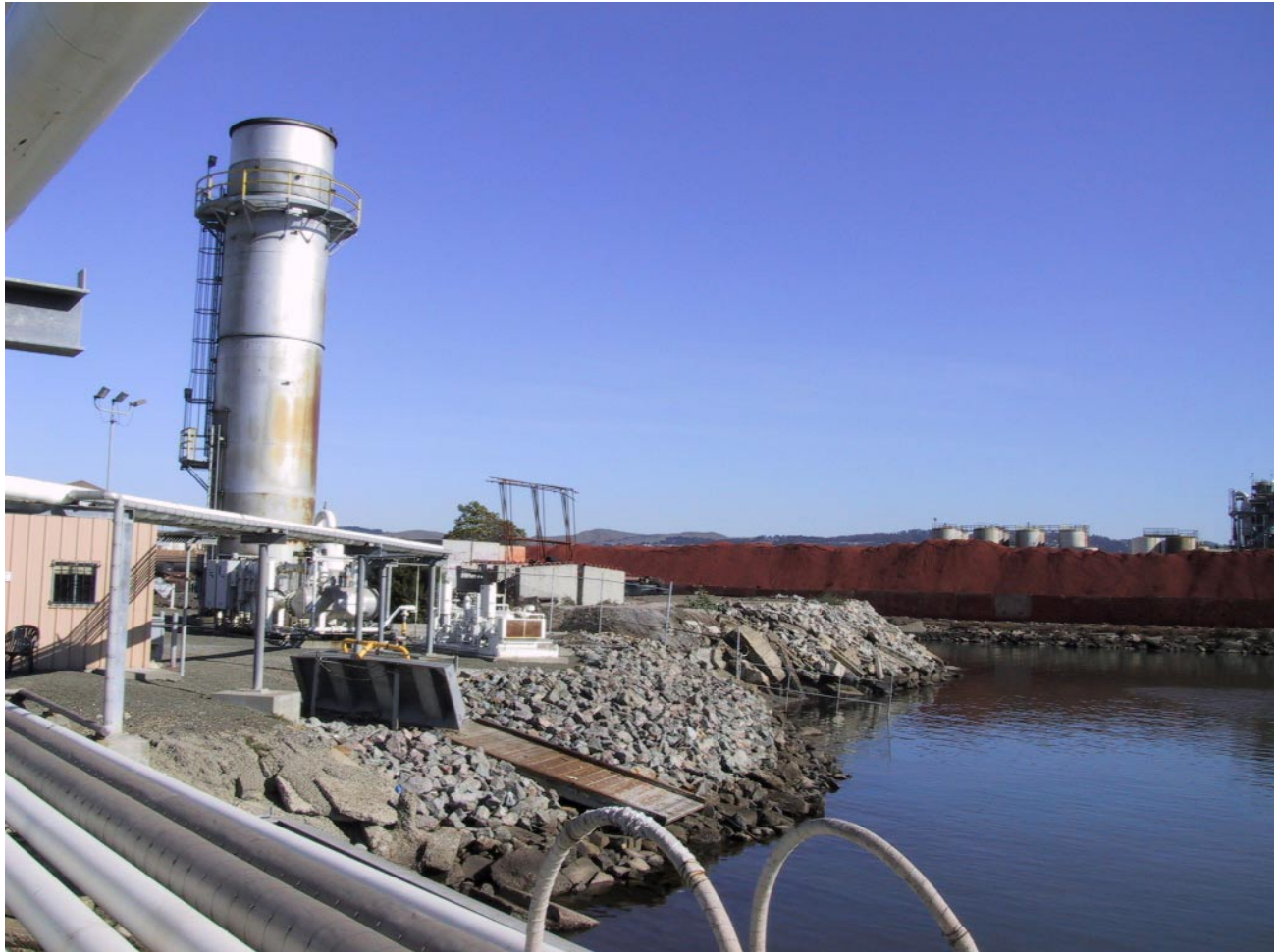
View of Eagle Rock aggregate storage site.
