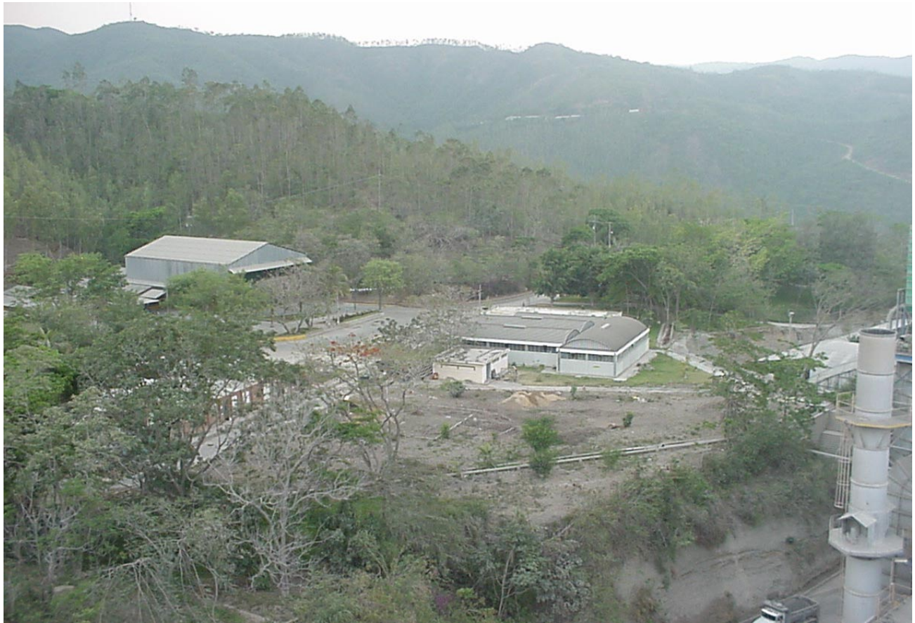
Overview of site location for clinker silo foundations.
