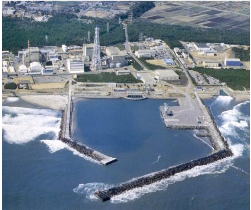
Aerial view of Tokai Nuclear Power Plant.
