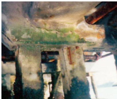
Conventional repair of piles and pilecap by dry-mix shotcreting.
