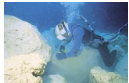
Underwater placement of boulders into reef.
