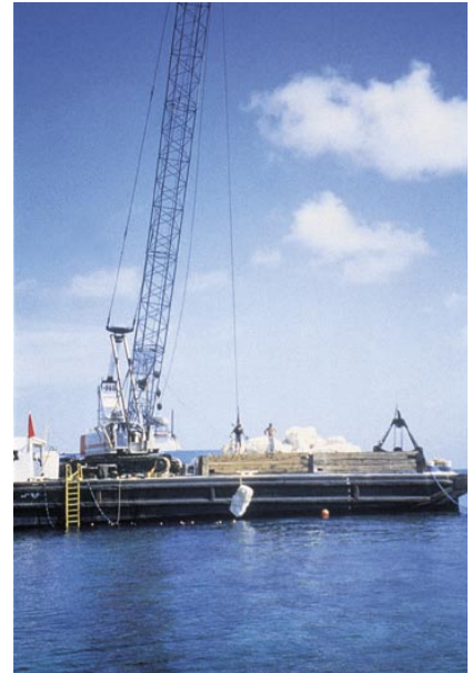
Placement of boulders from barge.
