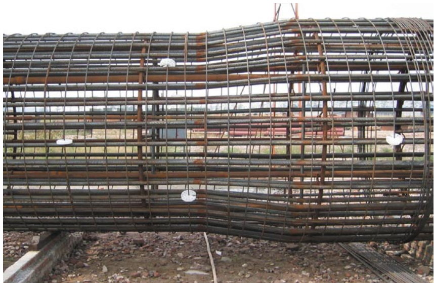
Drilled shaft casing.
