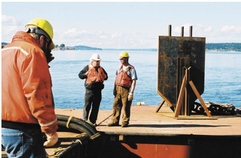
Installation of pile-driven plate anchor.
