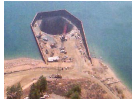
Aerial view of completed enclosure.
