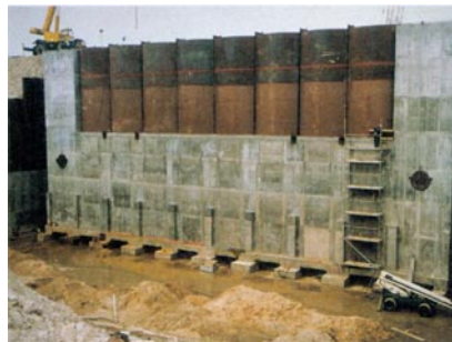
Excavation of enclosure behind float-in gate.
