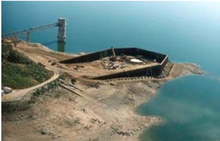
Construction of sheet-pile cofferdam enclosure.
