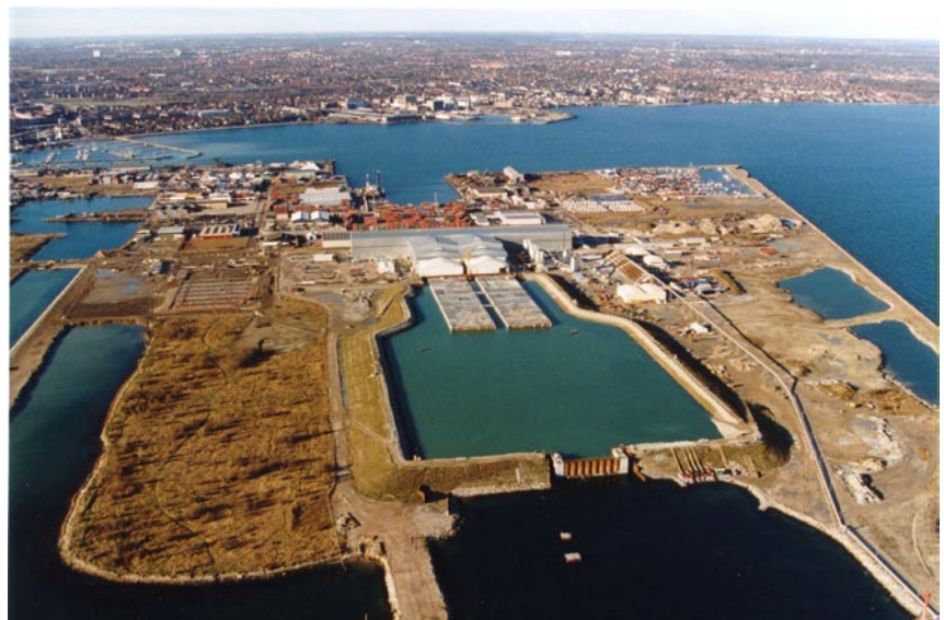
Casting yard enclosure prior to dewatering.
