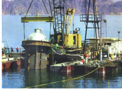
Installation of Intake Pipeline.
