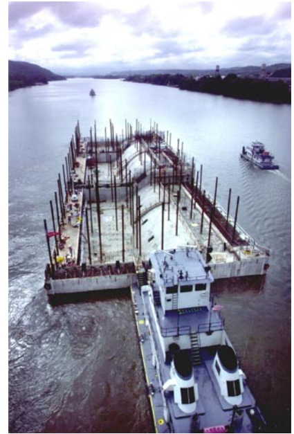
Float-in of concrete hull prefabricated offsite.
