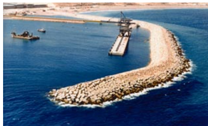
Puerto de Carboneras Breakwater, Spain.
