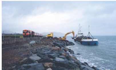
Coastal defense works on the Irish East Coast.
