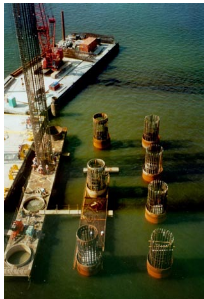
Installation of drilled shafts for the new Cooper River Bridge, Charleston, SC.
