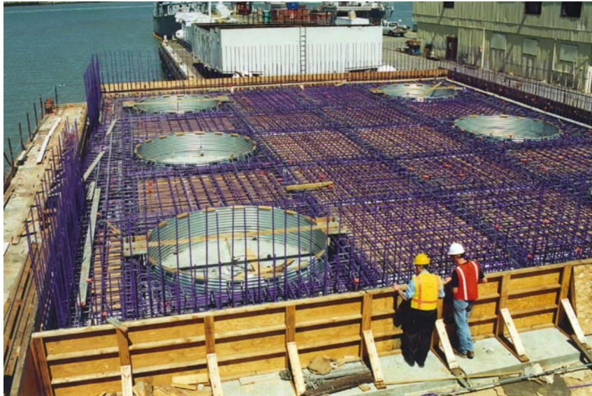
Casting of float-in cofferdam for Installation of drilled shafts for support of the four main tower legs of the New Carquinez Bridge, Crocket, CA.
