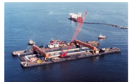
Catamaran barge for pre-cast shell deployment.
