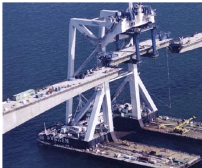
Heavy-lift catamaran barge, Svanen.
