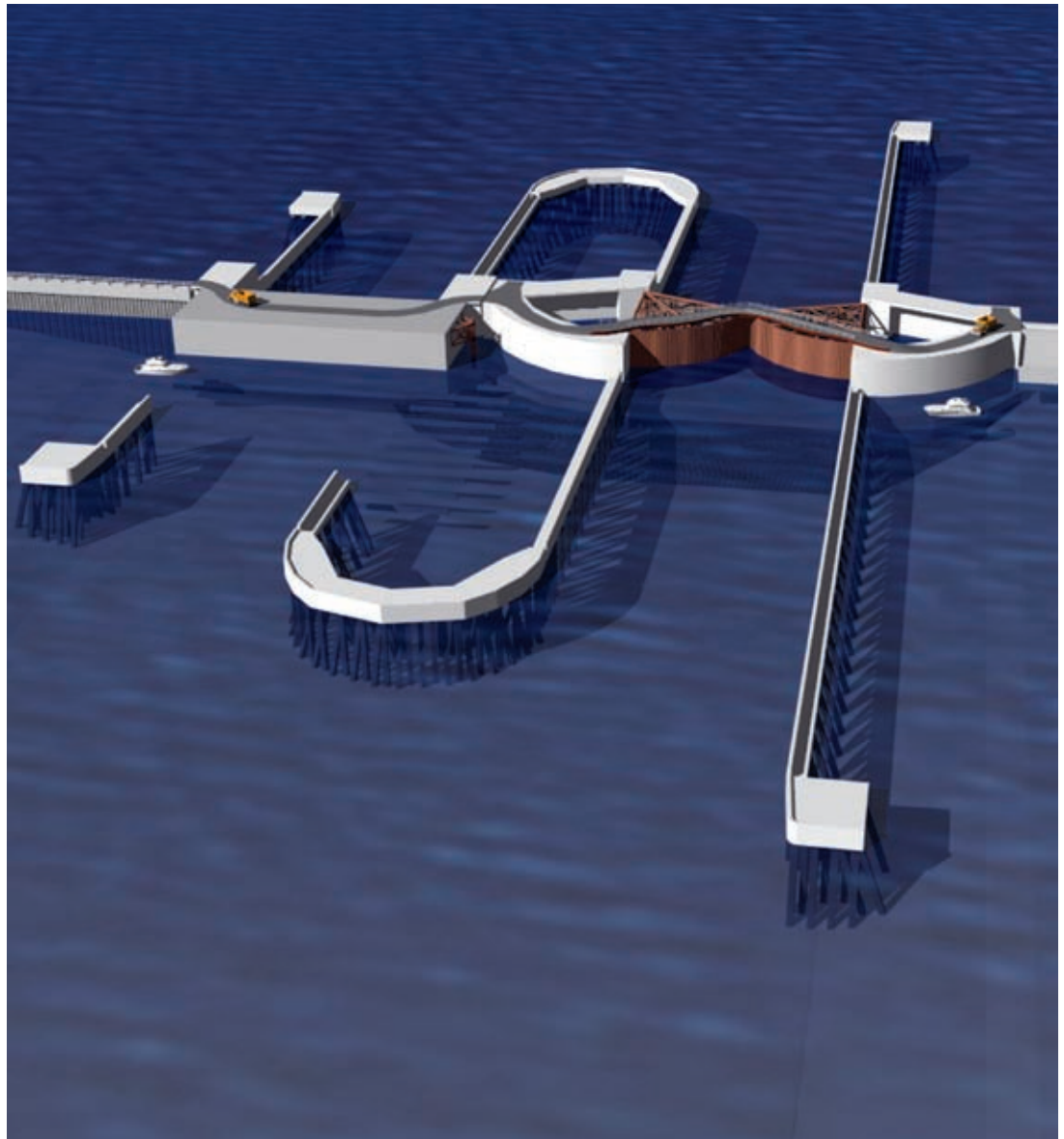
View of the GIWW Bypass and Sector Gate Structures for the IHNC Flood Protection Barrier
