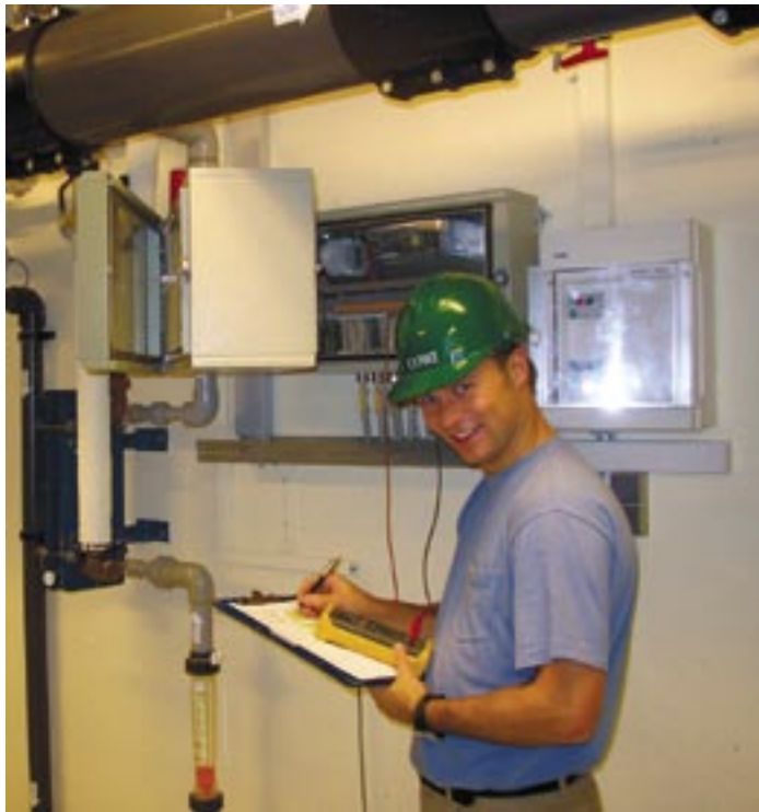
Service check-up of a cathodic protection installation in a swimming bath.
