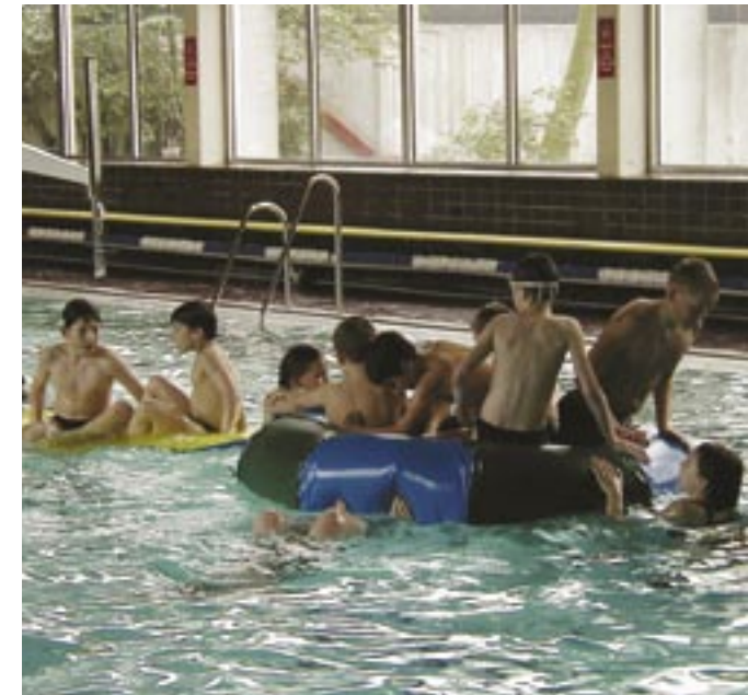
Engholm swimming bath - cathodic protection of pool structures and deteriorated deck sections.
