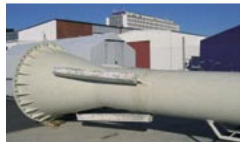
Säkrare Farleder Göteborg - cathodic protection with Aluminium sacrificial anodes in combination with surface coating extends the service life.
