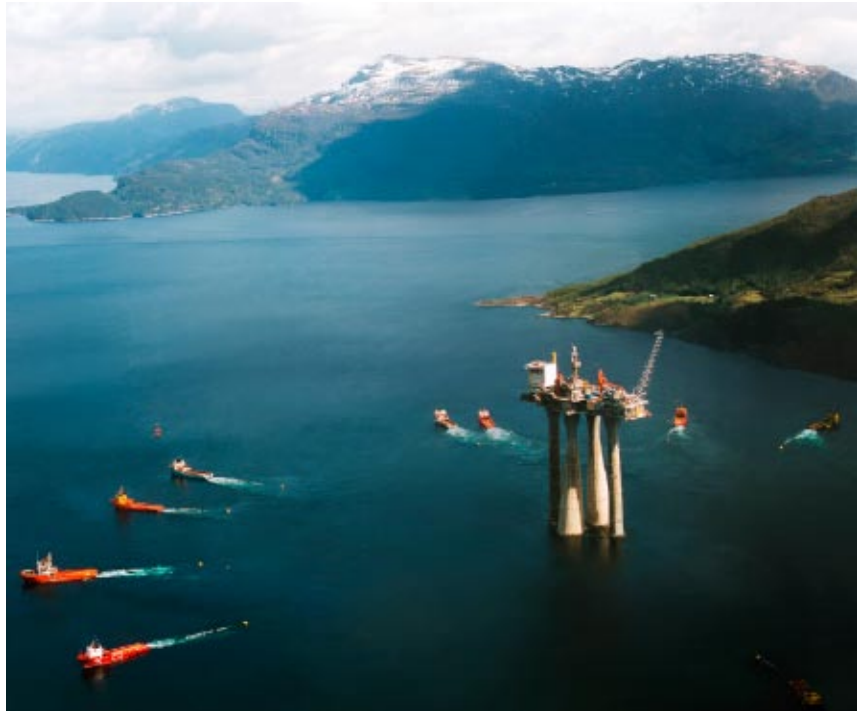
Tow-out of Troll East GBS Platform, Norway
