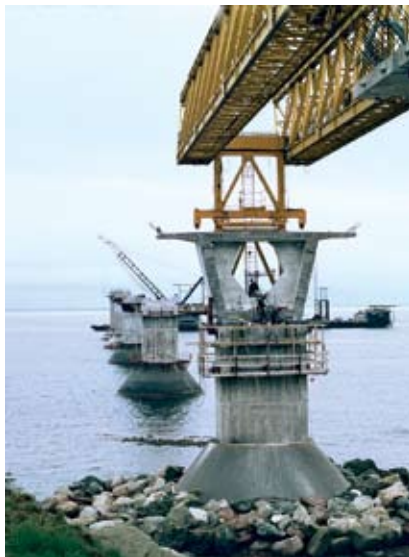
Confederation Bridge, Canada
