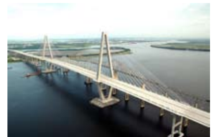
New Arthur Ravenel, Jr. Bridge across the Cooper River, Charleston, SC
