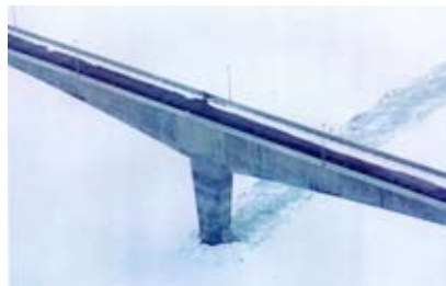
Ice loading on bridge piers, Confederation Bridge, Canada
