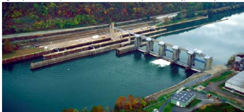
Charleroi Locks and Dam, Monongahela River, Pennsylvania
